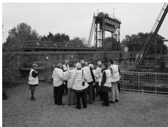
Project Manager Rob Barker explaining the Little Eye works
