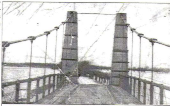
The original Suspension Bridge - Road still flooded!
