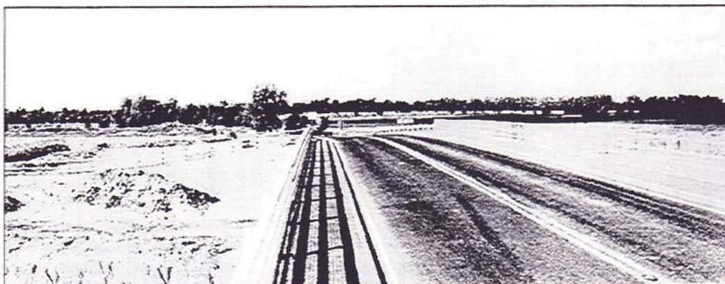
The Washes from the new 'Suspension' Bridge
